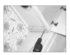
5. Reinforce cabinet base with 1x2 wood strips if additional strengthening is required. Unscrew and
